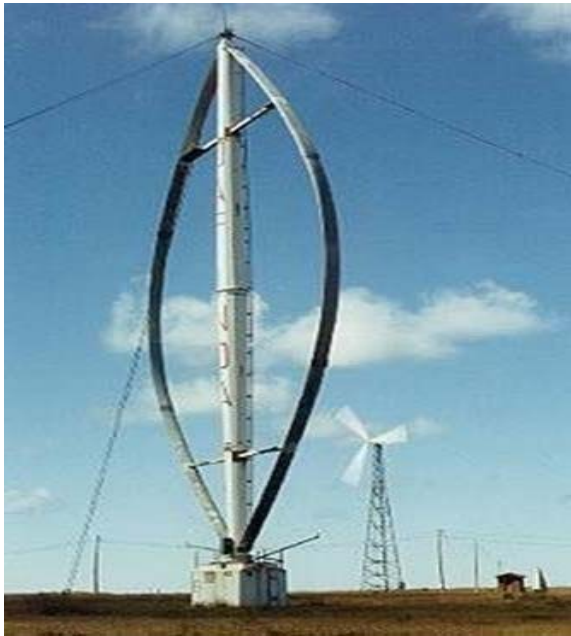
Figure-1. Darrieus vertical wind turbine with the generator positioned at the base of the tower. The tower is reinforced with guy wires.
